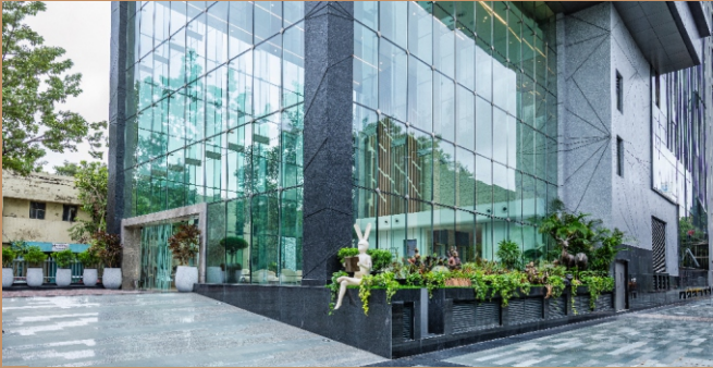
Contemporary façade with combination of stone, reflective heat-soaked glass & expanded metal screen
